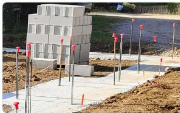
PHOTO Semelles filantes — ferrailage
